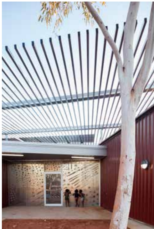
The Punmu Aboriginal Health Clinic in the Western Australian desert aimed to reinforce the organisational approach of respect of people, land and culture to create a facility with community ownership Photo courtesy Kaunitz Yeung
